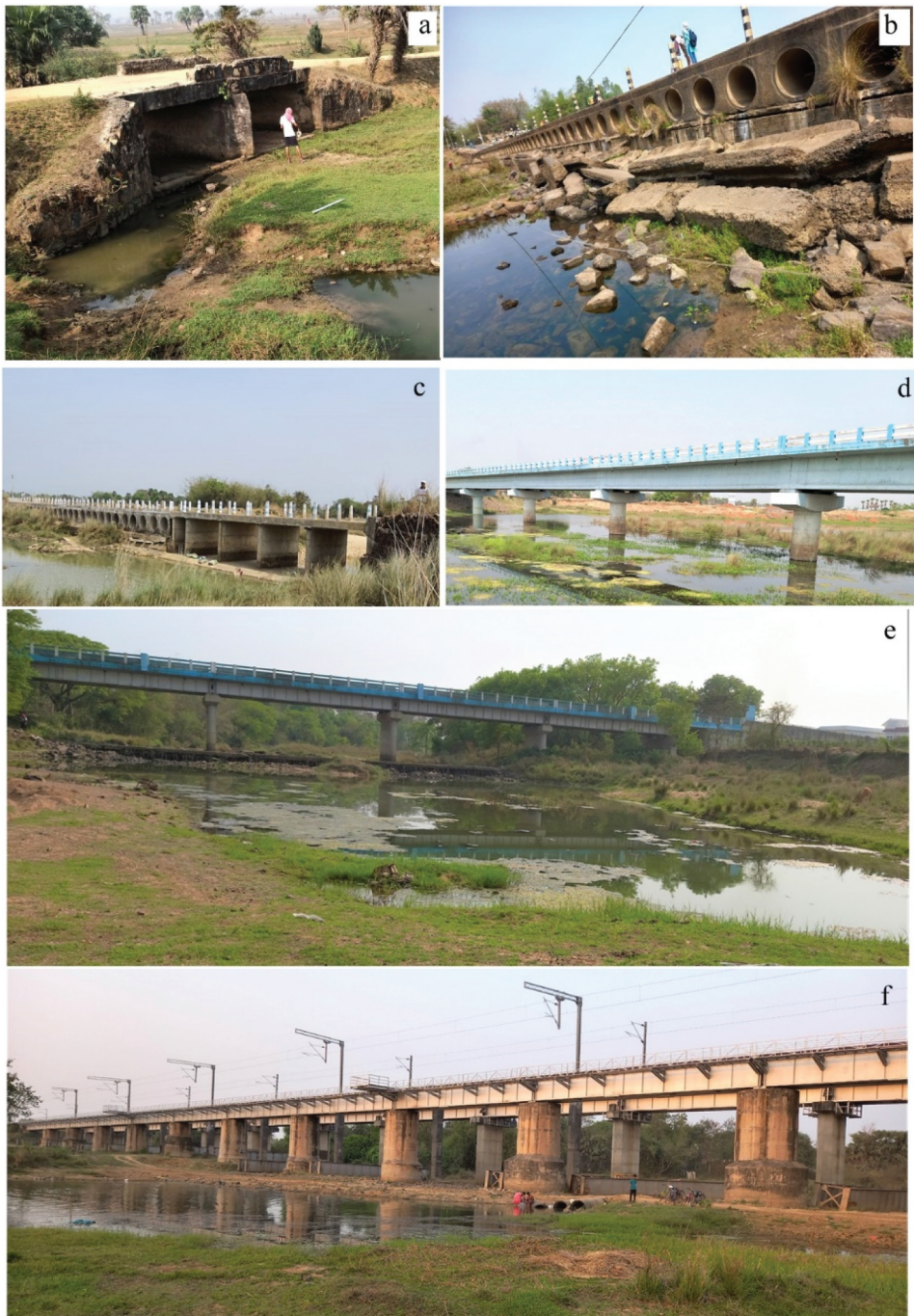
Figure 8. Different types of piers and their locations observed on the Kopai River: a. Box nose piers near Khajuri, b. Round nose piers near Chandipur, c. Mixed nose (round and box) near Galtia, d. Cylinder nose piers near Adityapur, e. Nose piers near Ballavpur, f. Cylindrical and Sharp nose piers near Taltor Prantik rail bridge crossings.
