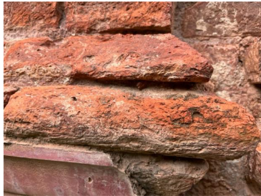
Fig. 2. Corroded brick.
