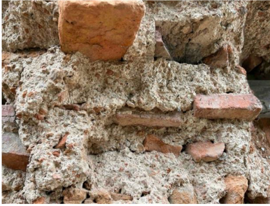
Fig. 3. Corroded plaster.
