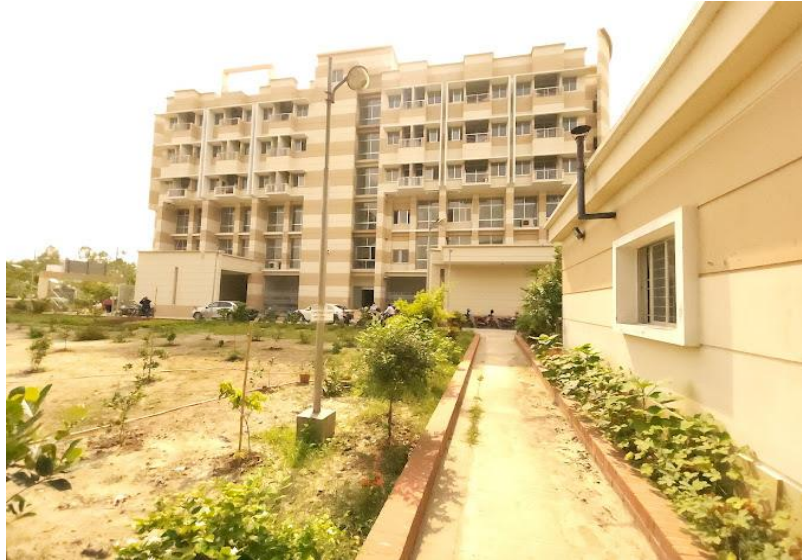
Figure 1: Building of Munshiganj Diabetes Hospital
