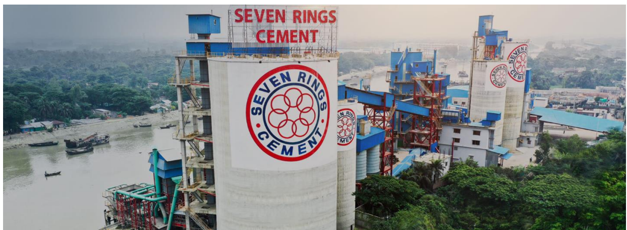
Fig 2 : Seven Rings Cement Company.
