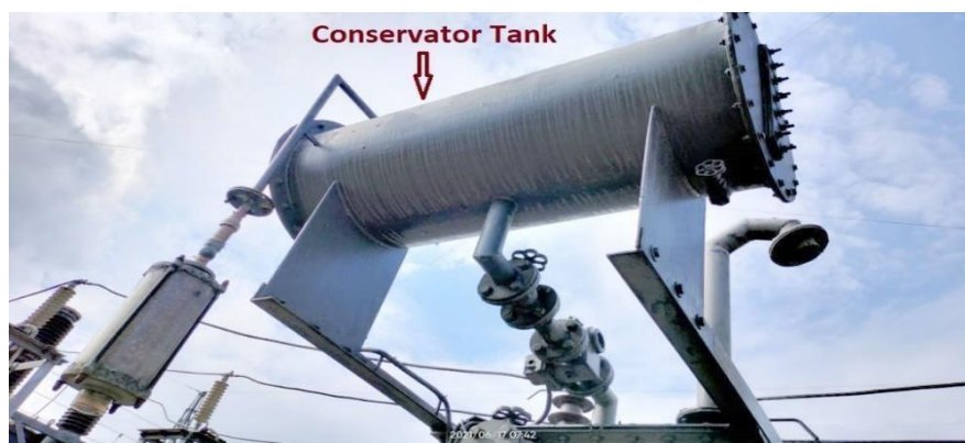
Figure 5.2: Conservator Tank.
