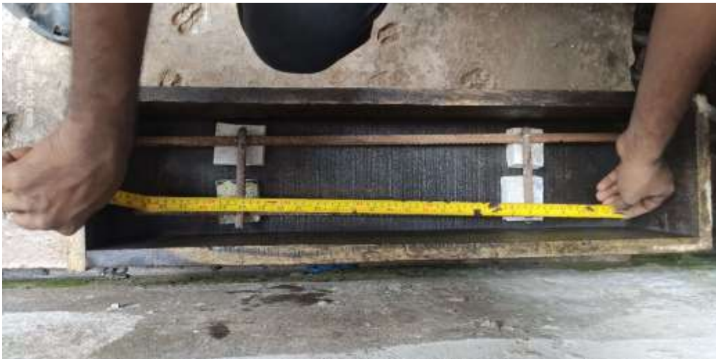
Figure 3.9.1: Formwork setup
