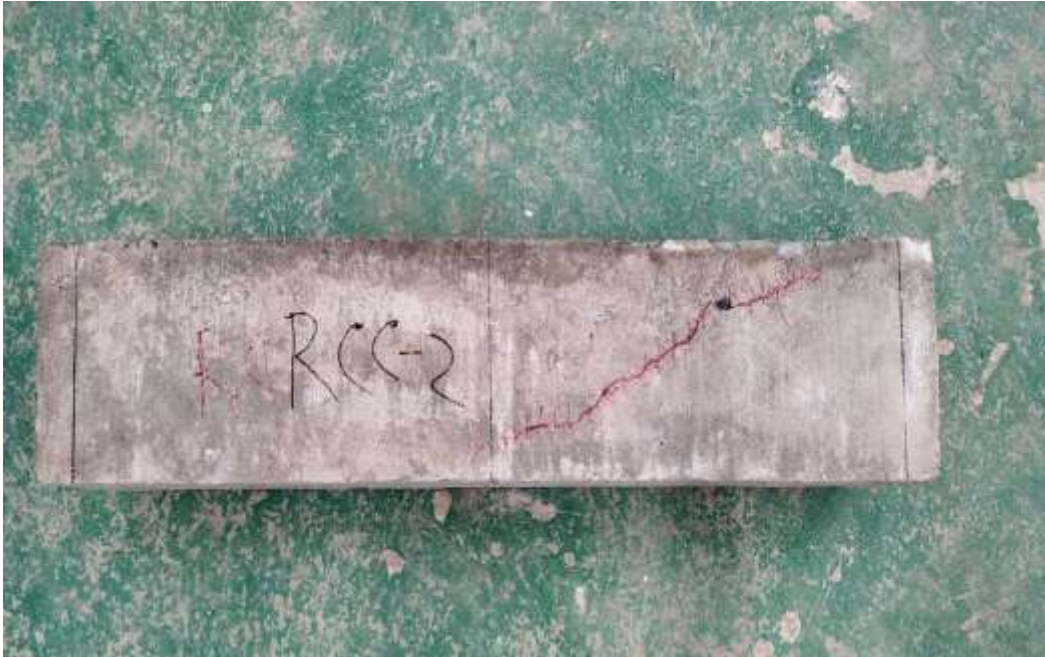
Figure 4.8.5: Failure Pattern (for Type 2-2 Beam)
