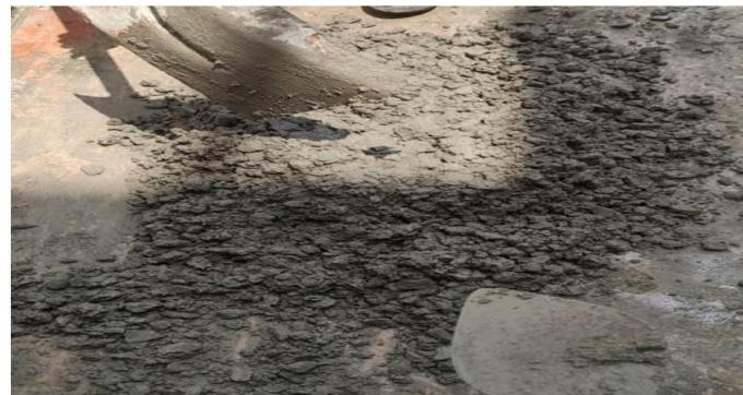
Figure 3-6: Wet concrete mix
