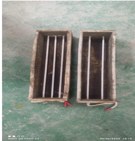
Figure 3-11: Formwork of beam
