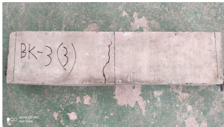
Figure 4-43: Failure pattern (Polyester fiber beam)
