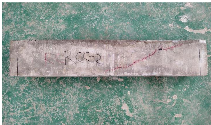
Figure 4-8: Failure pattern (Reinforcement beam)
