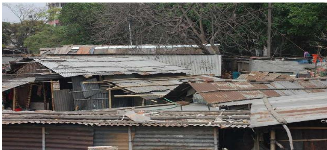
Fig.2.2 The state of housing in the Chalantika community
