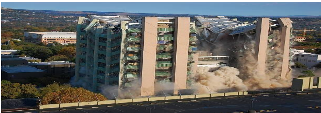
Fig. 3.1: Deconstruction by implosion method
