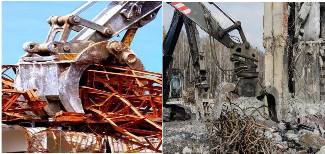
Fig. 3.12: Metal recycling process
