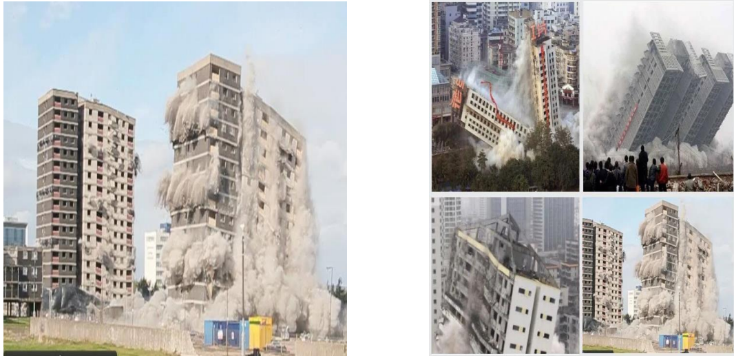
Fig. 3.2: Implosion method using dynamite
