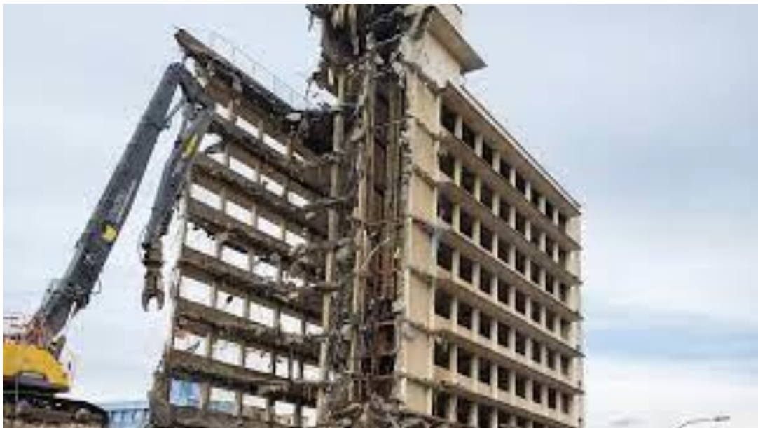
Fig. 3.6: Hydraulic excavator joints with steel pusher arm
