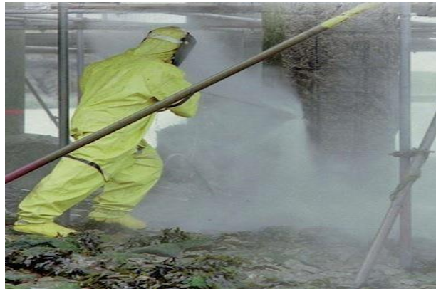
Fig. 3.9: Pressure or hydro-demolition
