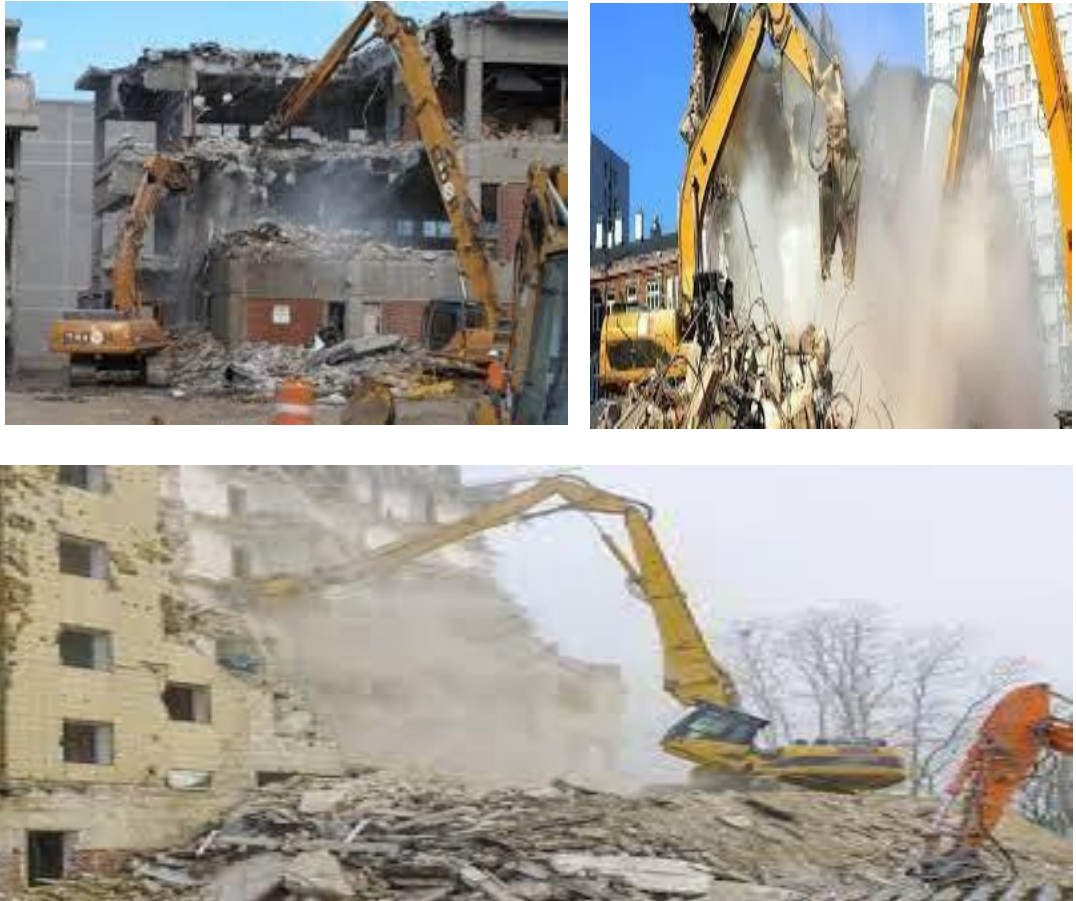
Fig. 3.7: Pusher arm demolition techniques
