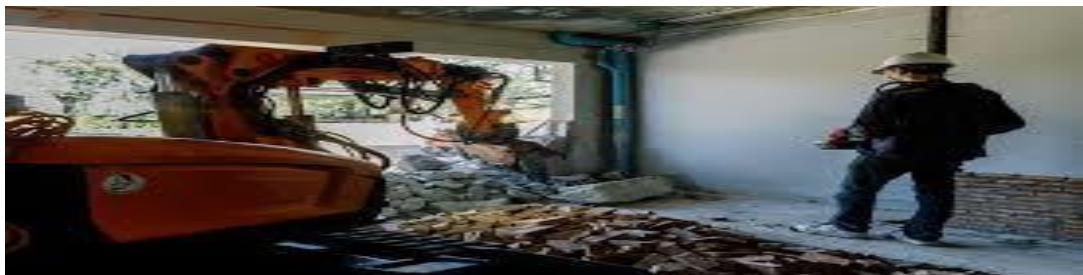
Fig. 3.17: Remote controlled machinery
