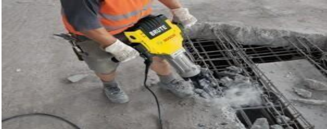
Fig. 3.5: Manual method using breaker hammer
