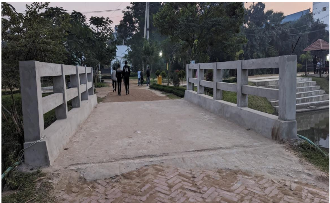
Fig. 1.2 View of the DIU lake bridge
