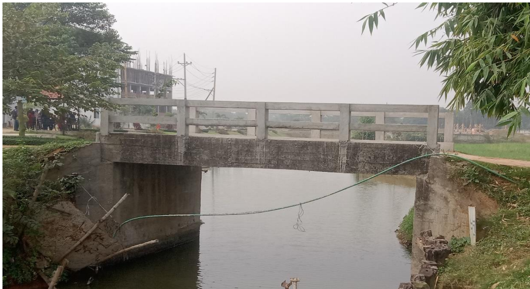
Fig. 1.4 DIU lake bridge west side
