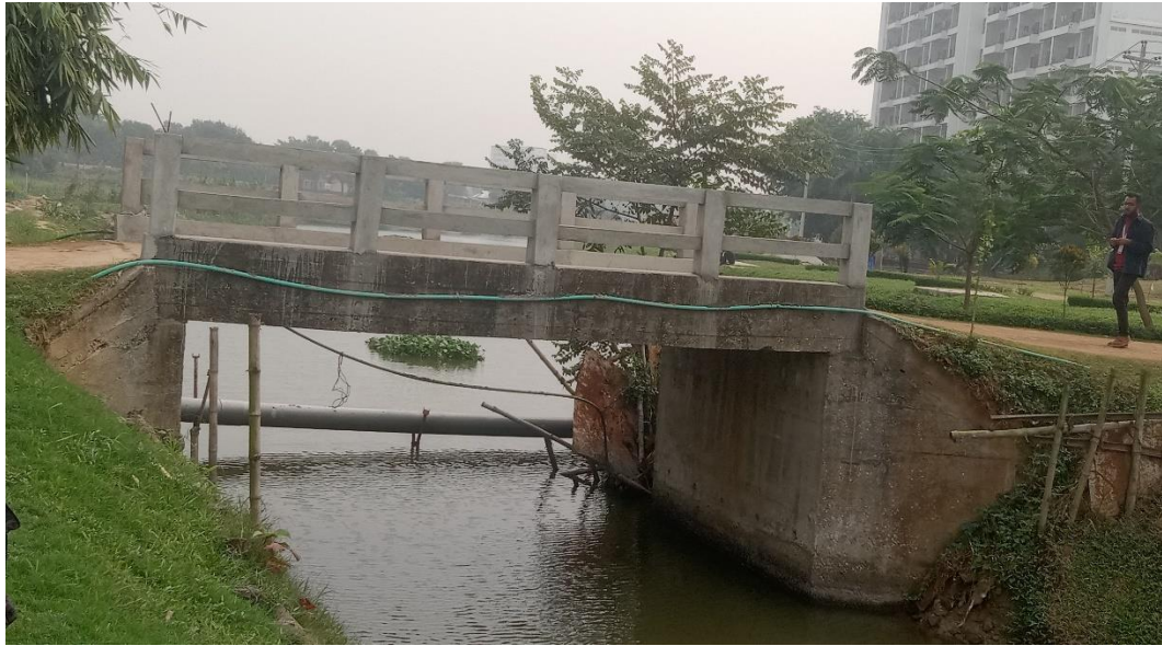
Fig. 1.3 DIU lake bridge east side
