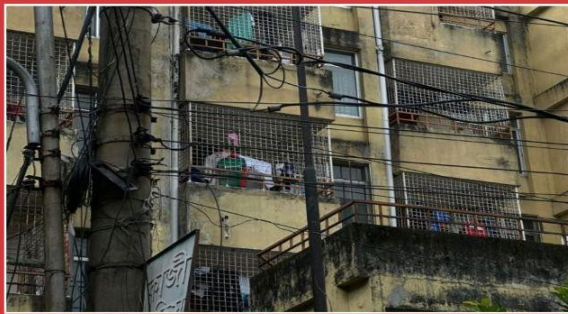
Exterior shot of the building
