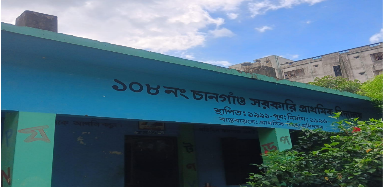
Image Of 108 No. Changaon Govt. Primary School.
