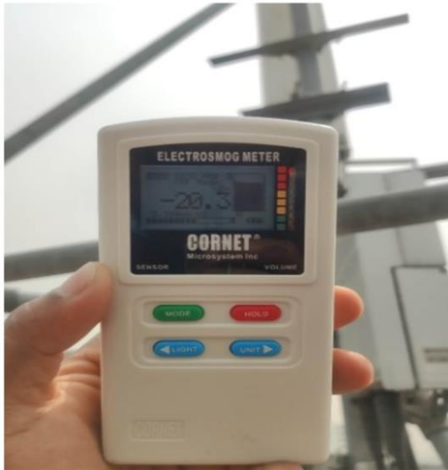
(Radiation from BTS Antenna)
