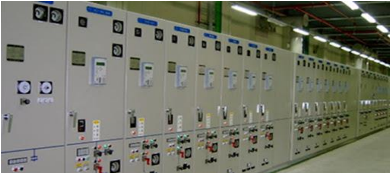
Figure 4:1 Switchgear
