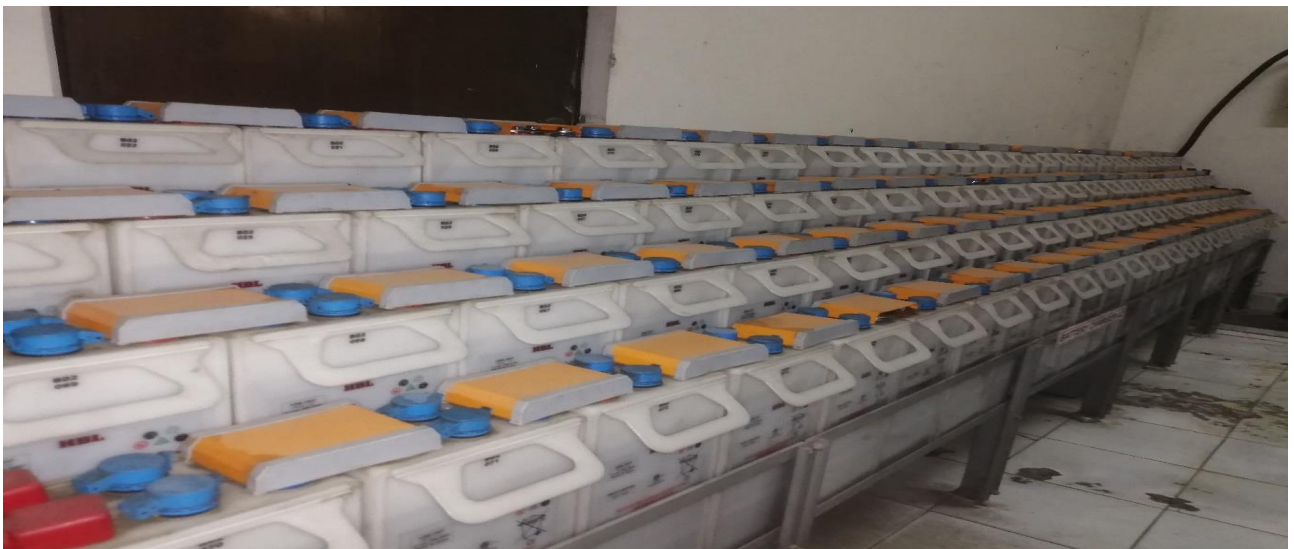
Figure 6:7 Back-up (Battery)
