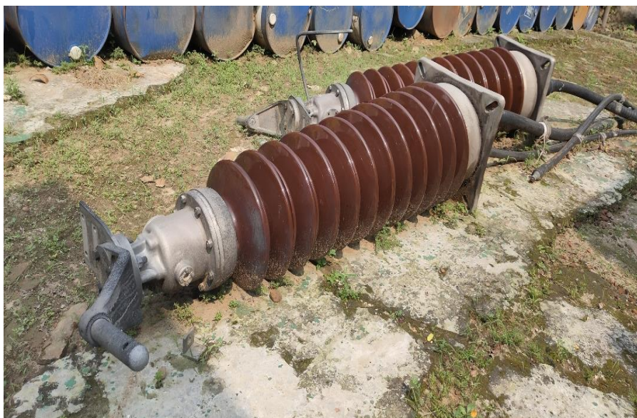
Figure 6:4 Lightning Arrester
