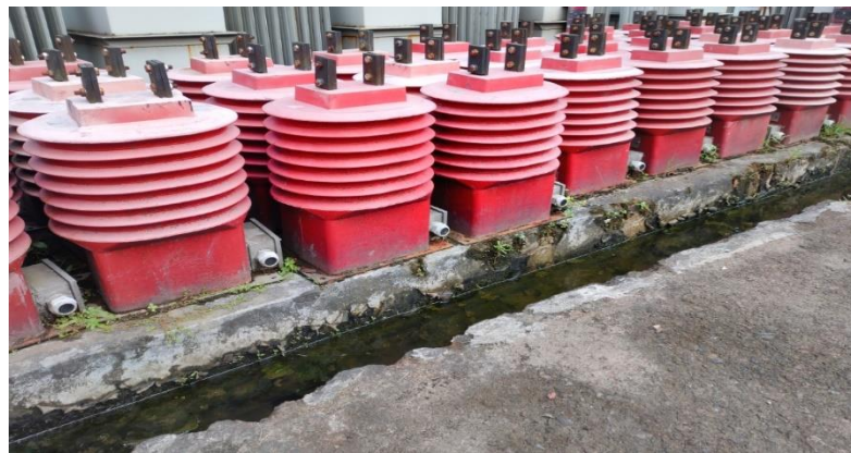
Figure 6:1 Current transformer
