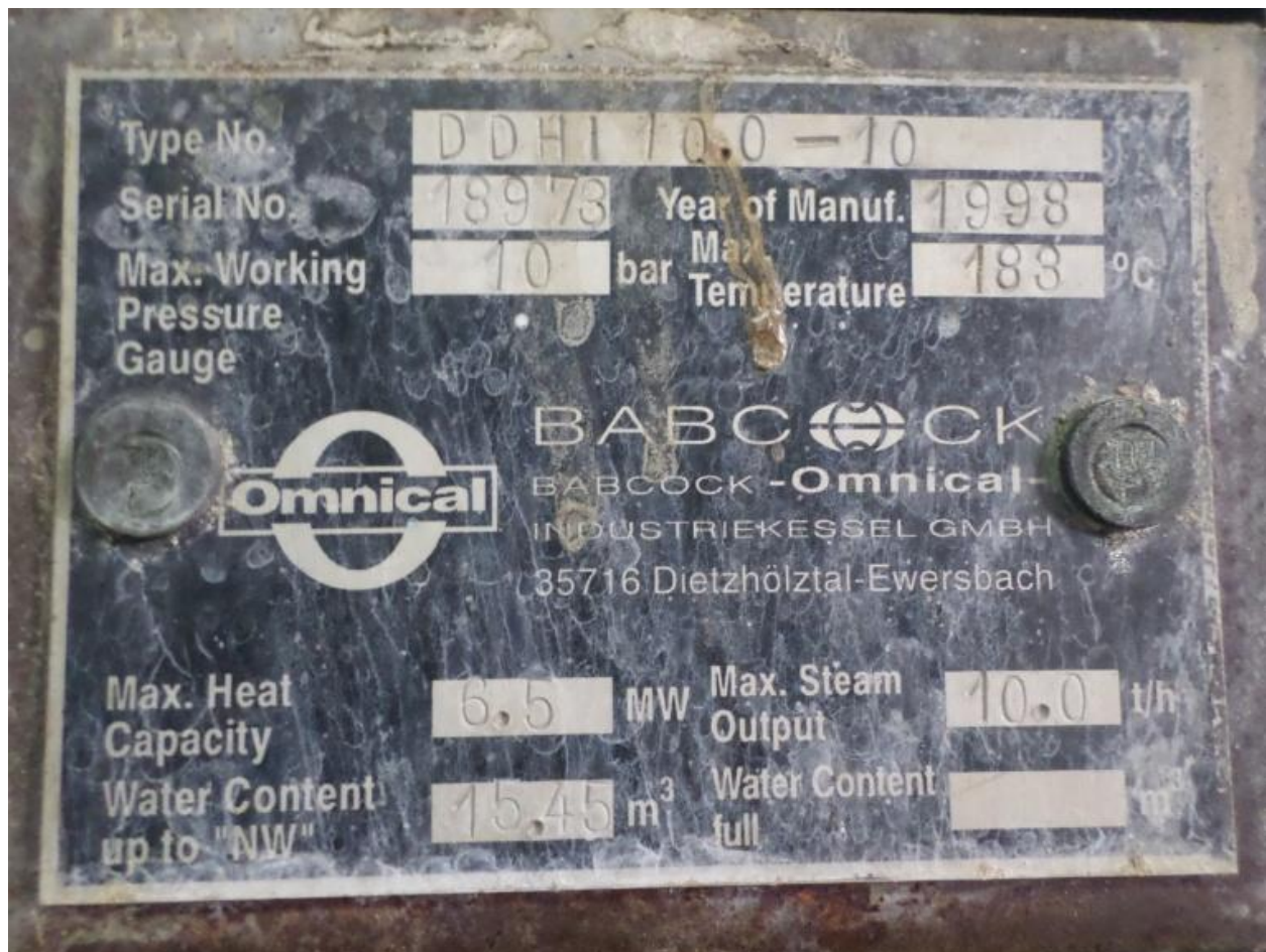
Figure: Specification of boiler used in Shasha Denims Ltd.
