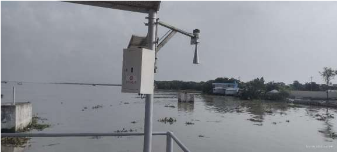
Figure 3.3.11: River Surface level monitoring station.
