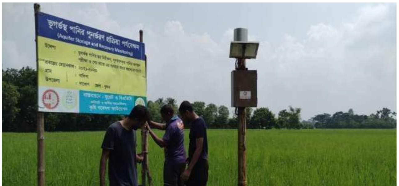
Figure 3.3.4: Groundwater level monitoring station setup on field.
