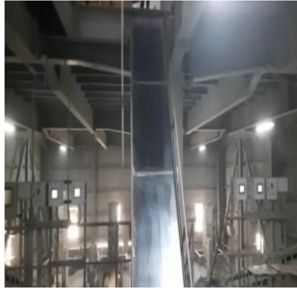
Figure-41: After Chute Making
