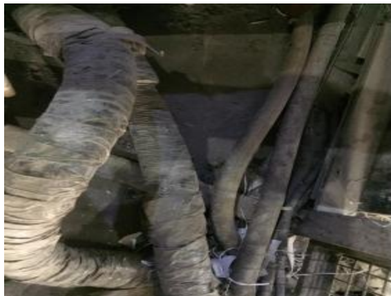
Figure-27: Before motor Installation
