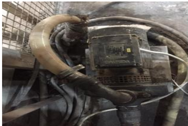
Figure-28: After Motor Installation
