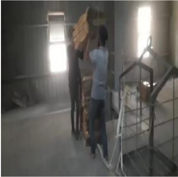
Figure-40: Before Chute Making
