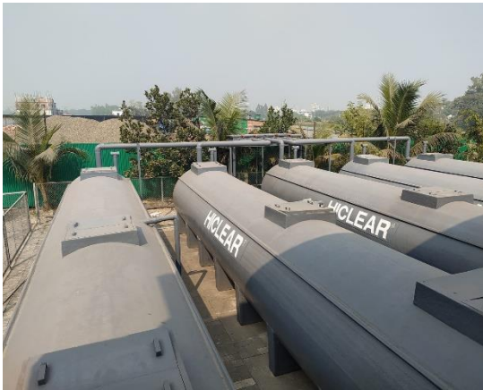
Figure 3.4.3: STP Chamber
