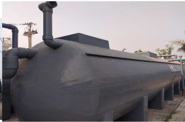
Figure 3.4.2: STP Chamber
