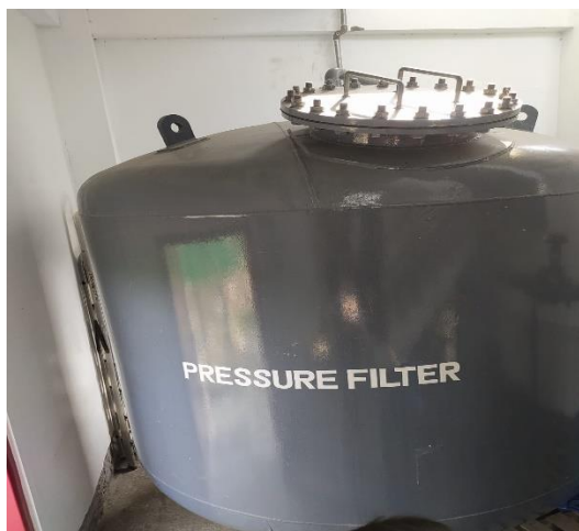
Figure 3.4.5: Pressure Filter
