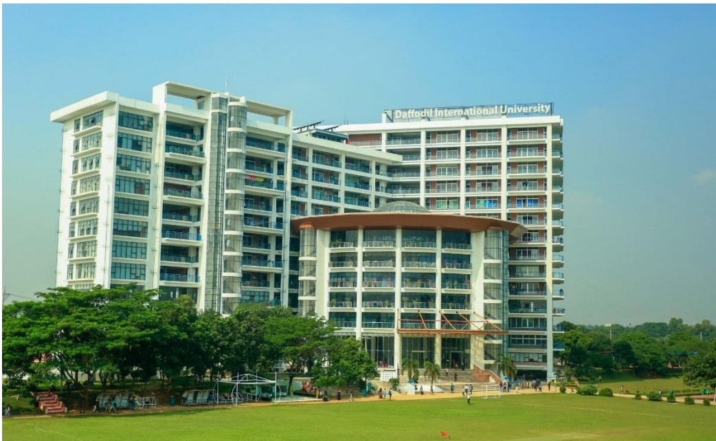
Figure 11.3: AB4 Building Reference
