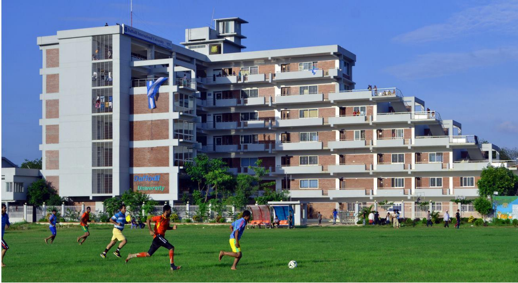
Figure 11.2: AB Building Reference
