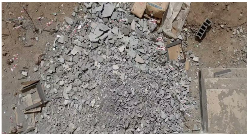
Figure 3. 2: Broken Parking Tiles (Sample)
