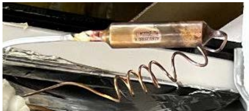
Fig. 3.5 Capillary tube and filter driver
