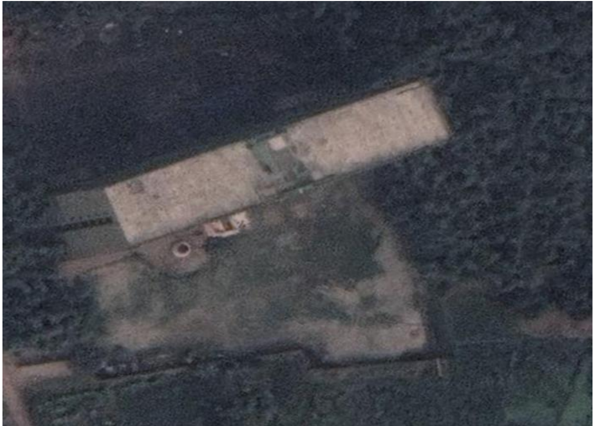
Figure 3.3: Rooftop of YKSG-2 (Hall)
