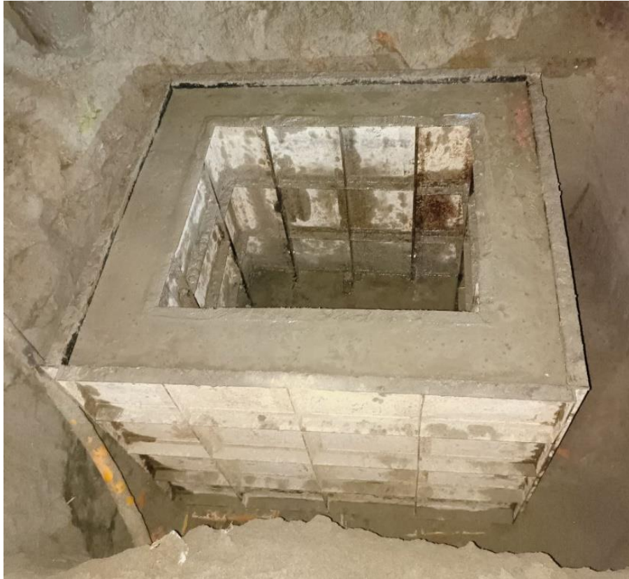
Image 3.2: HH Construction of SComm
