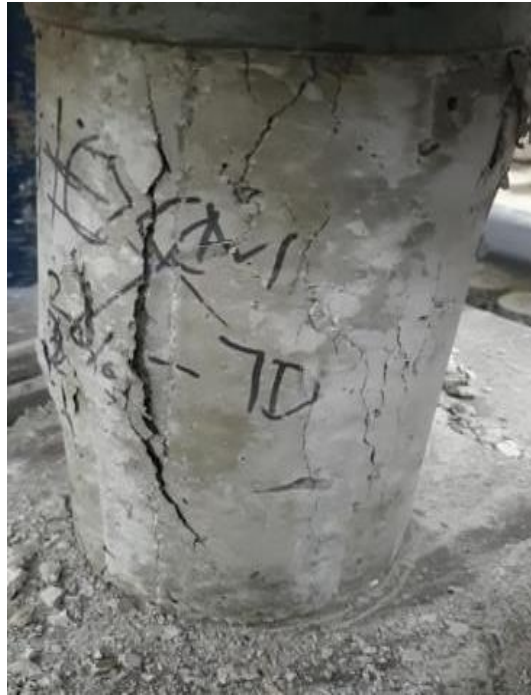
Fig 4.8: Concrete under compression Load
