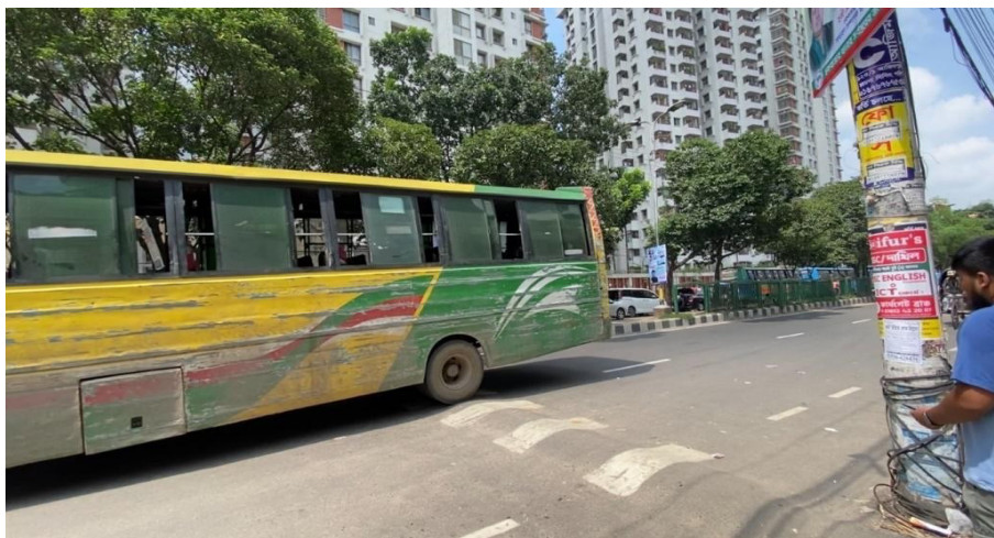
Figure 3.8: New Market back side Midpoint Speed Breaker,
