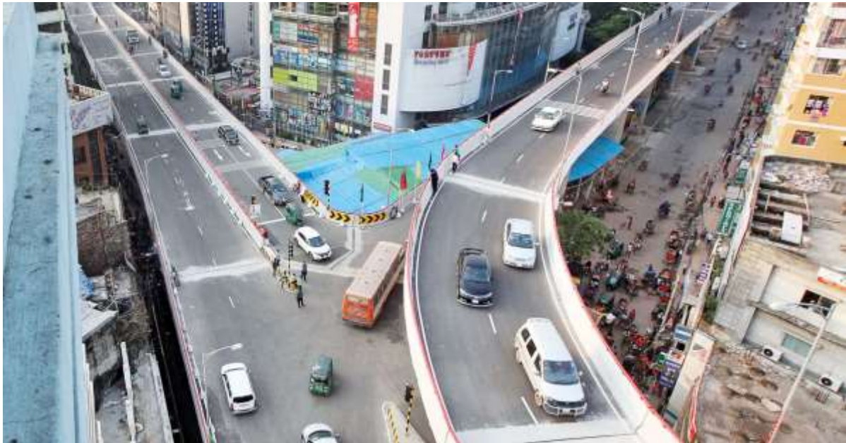
Figure 1.1: Flyover infrastructure upgrades in major cities
