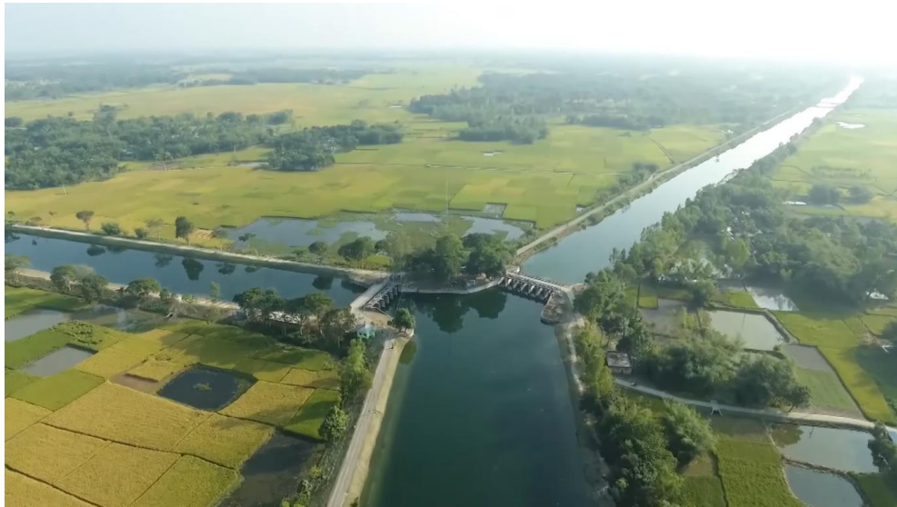
Figure 3.12: Teesta Barrage Area Water Distribution System
