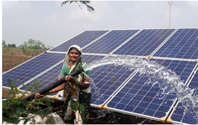
Figure 3.13: Solar Pumping Irrigation in Village [32]
