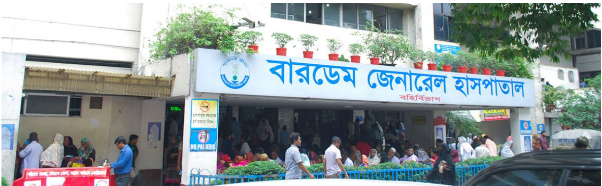
Figure 2: Entry point of BIRDEM
