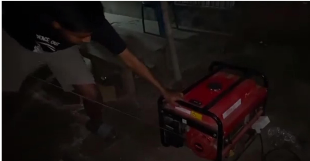
Figure 5.4: Turning on generator
