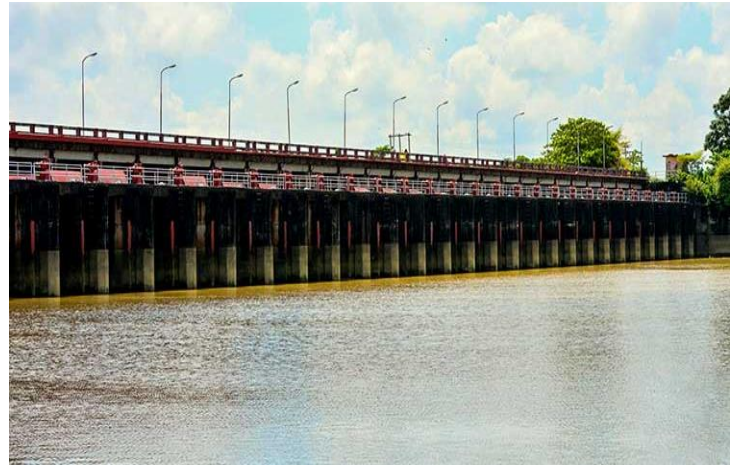
Fig 1.1: Muhuri Dam, Feni [4]
