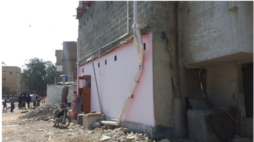
Fig. 2 Brightly coloured wall of one of the rebuilt structure
