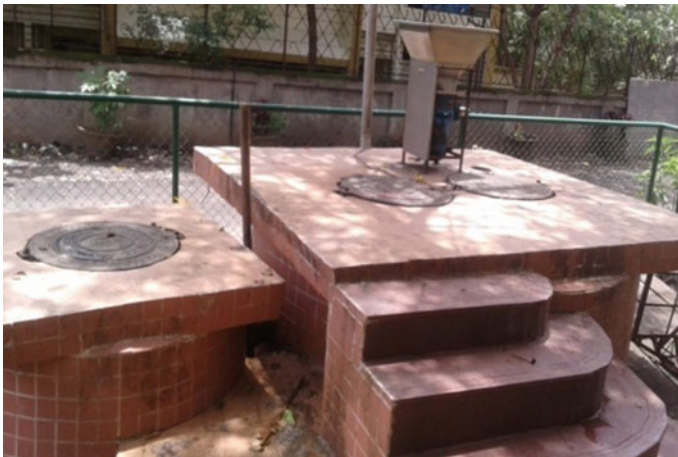
Fig. 4 Shredder above pre-digester
