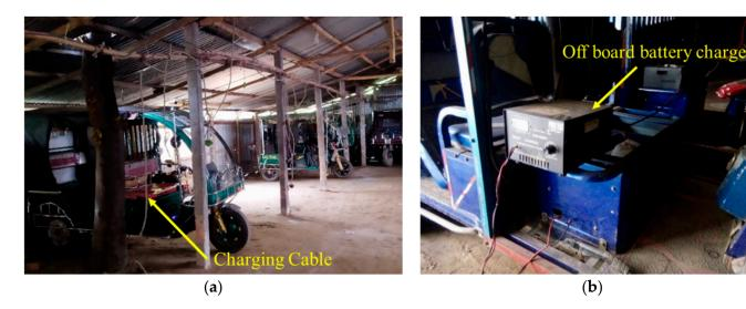
Figure 5. E3W charging station: (a) parking arrangement; (b) E3W charging.
