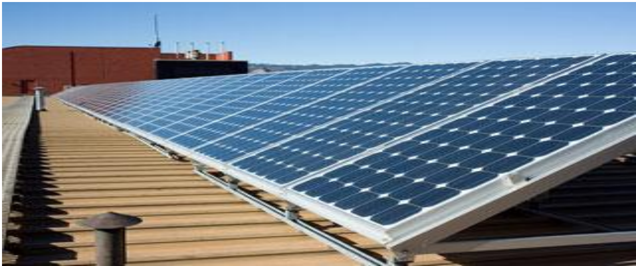
Figure 2.18. Angle Mounting on roof
