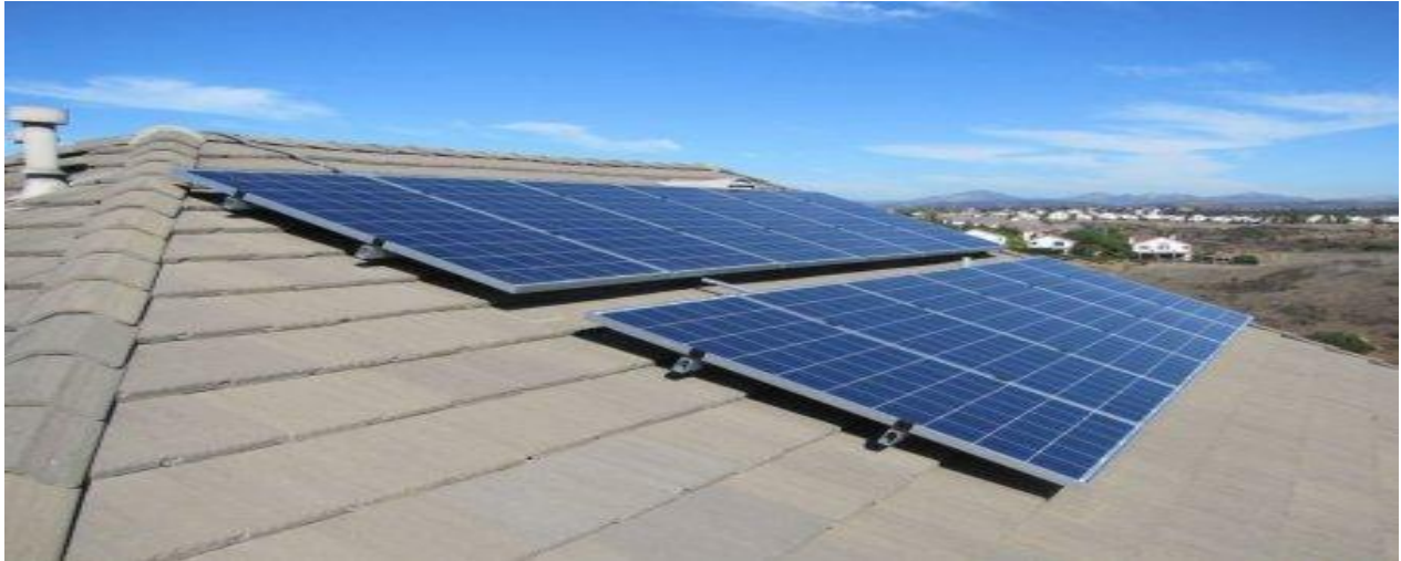
Figure 2.17. Flush Mounting on roof
