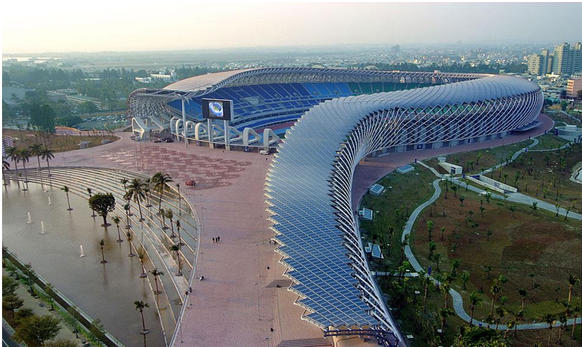
Figure 2.5: 100% Solar power stadium taiwan
