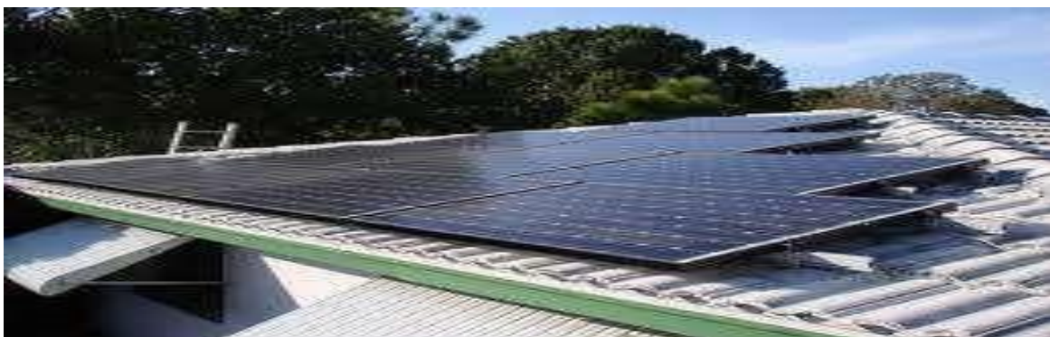
Figure 2.9.c: Fin mounting on roof
