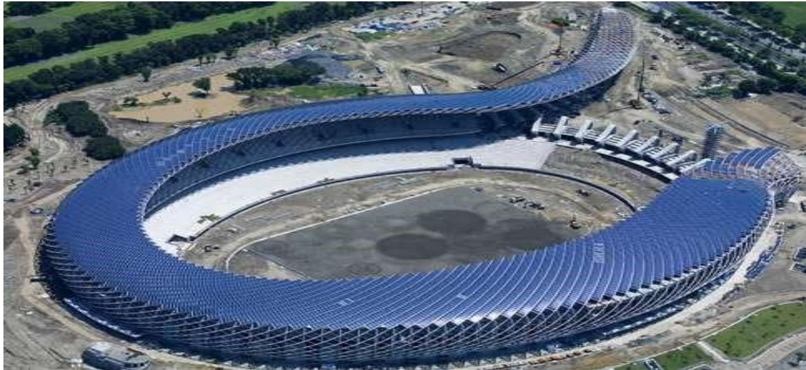
Figure 2.2.b. 100% solar powered stadium in Taiwan.
