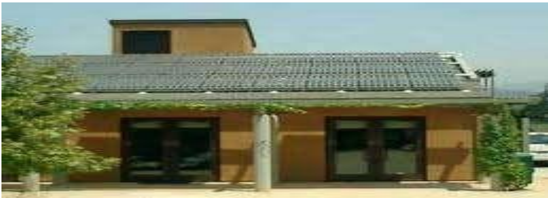
Figure2.9.b: Angle Mounting on roof
