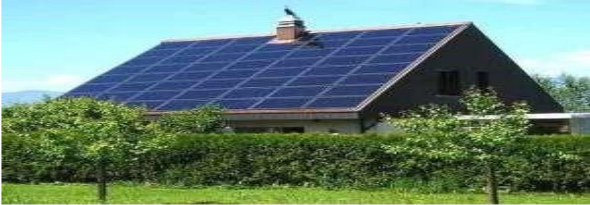
Figure 2.9.a.: Flush Mounting on roof
