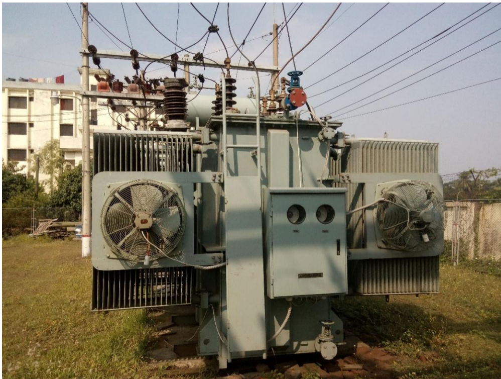
Fig. 2.5: Transformer with cooling system
