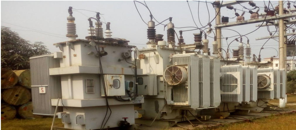
Fig. 2.1: Power Transformer
