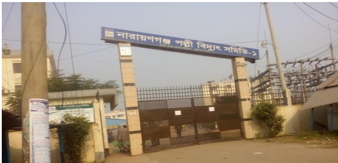
Fig. 1.1: Main gate of NPBS-1
