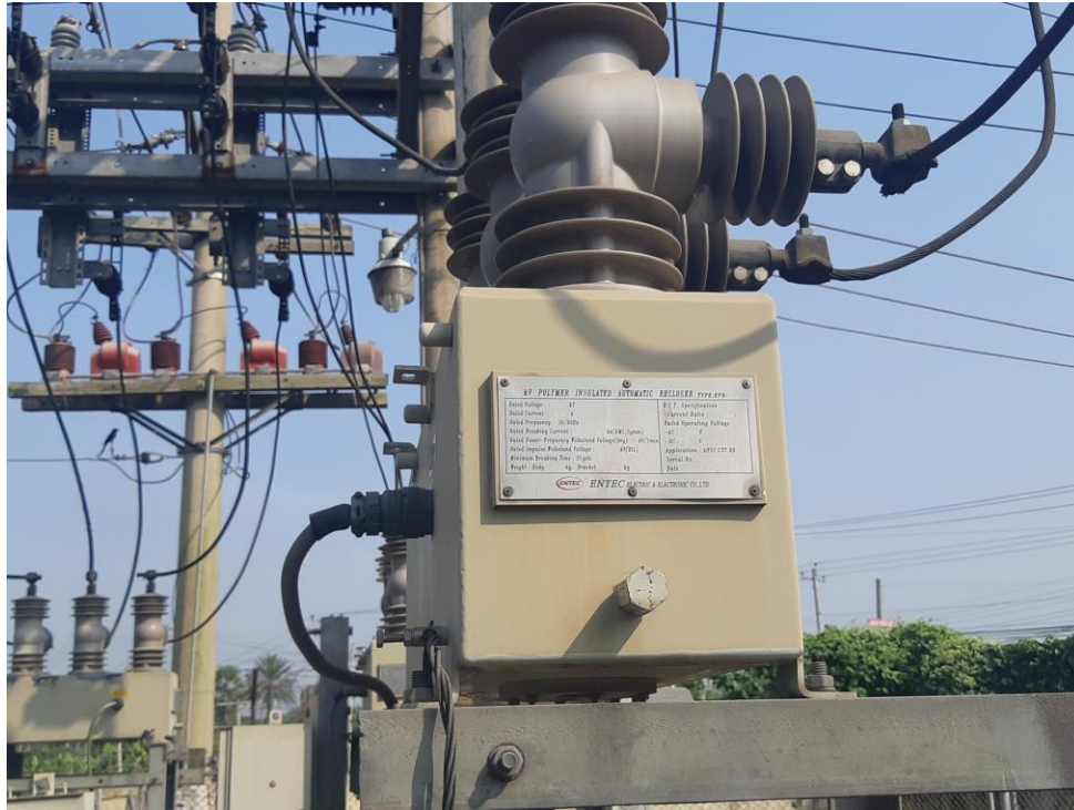
Figure 3.4: ACR of Narrayanganj PBS-1 Sub-Station
