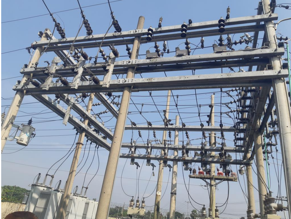
Figure 4.1: Bus-Bar Arrangement of Narayanganj PBS-1
