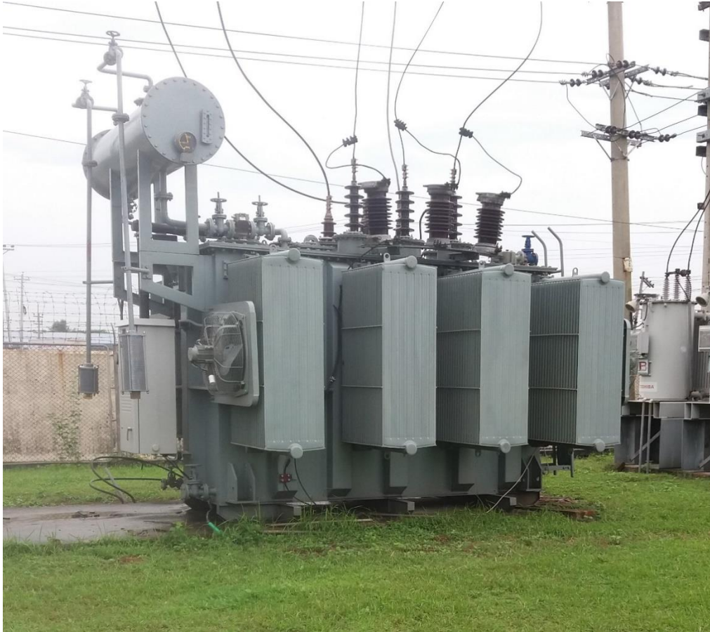
Figure 3.1: Power Transformer of Narayanganj PBS-1
