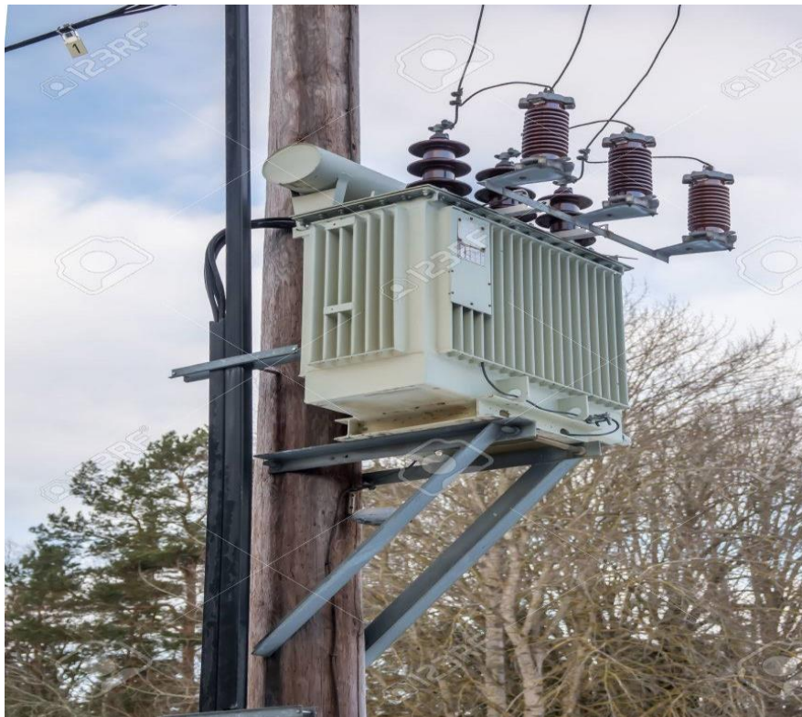
Figure 5.1: Distribution Transformer
