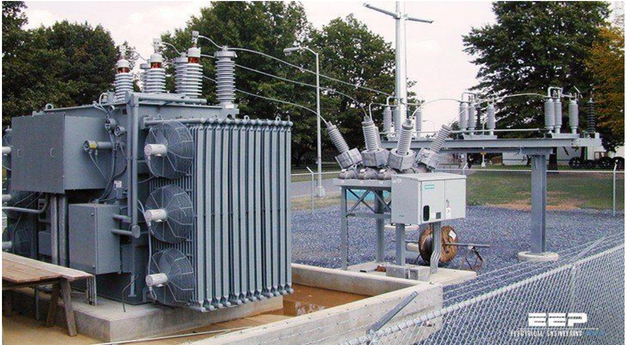
Fig 3.3: Oil Transformer
