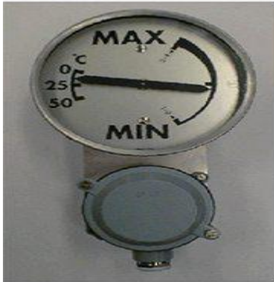
Fig 3.10: A typical outlook of an oil level monitor device
