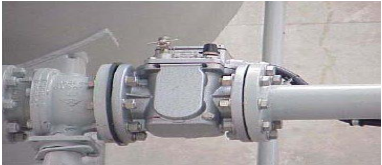
Fig 3.4: Installed Buchholz gas relay
