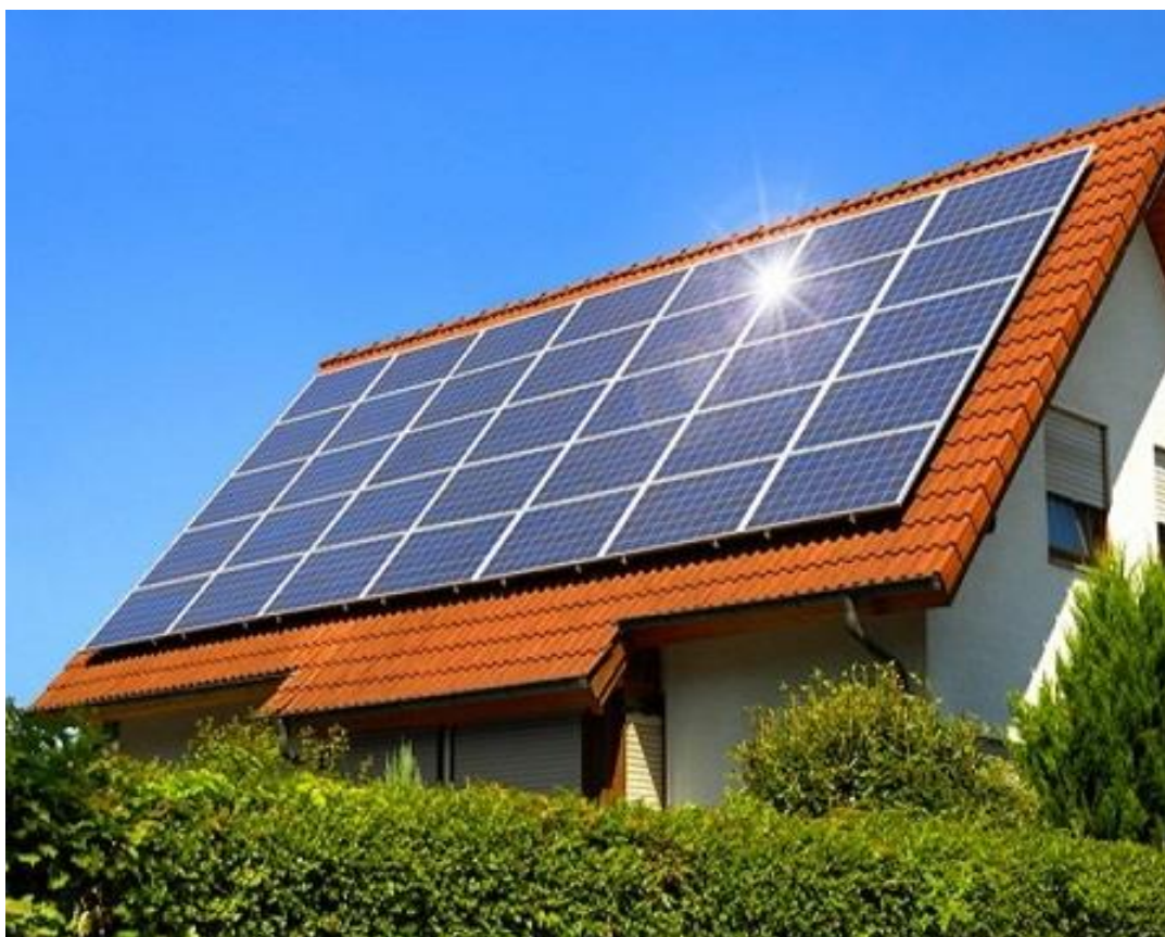
Fog: 2.11 Solar Rooftop System
