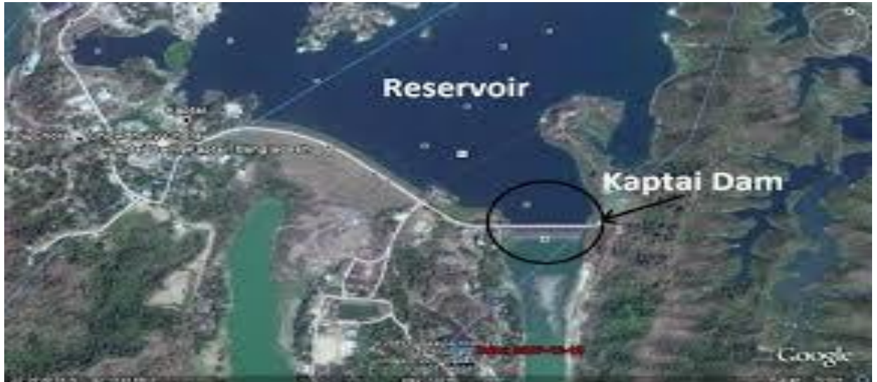
Fig: 2.4 Satellite view of Karna fully hydropower plant
