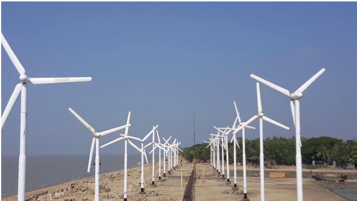
Fig-2.1: wind power plant
