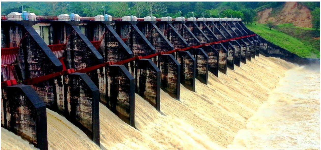
Figure 2.3 Hydroelectric Power plant in Kaptai
