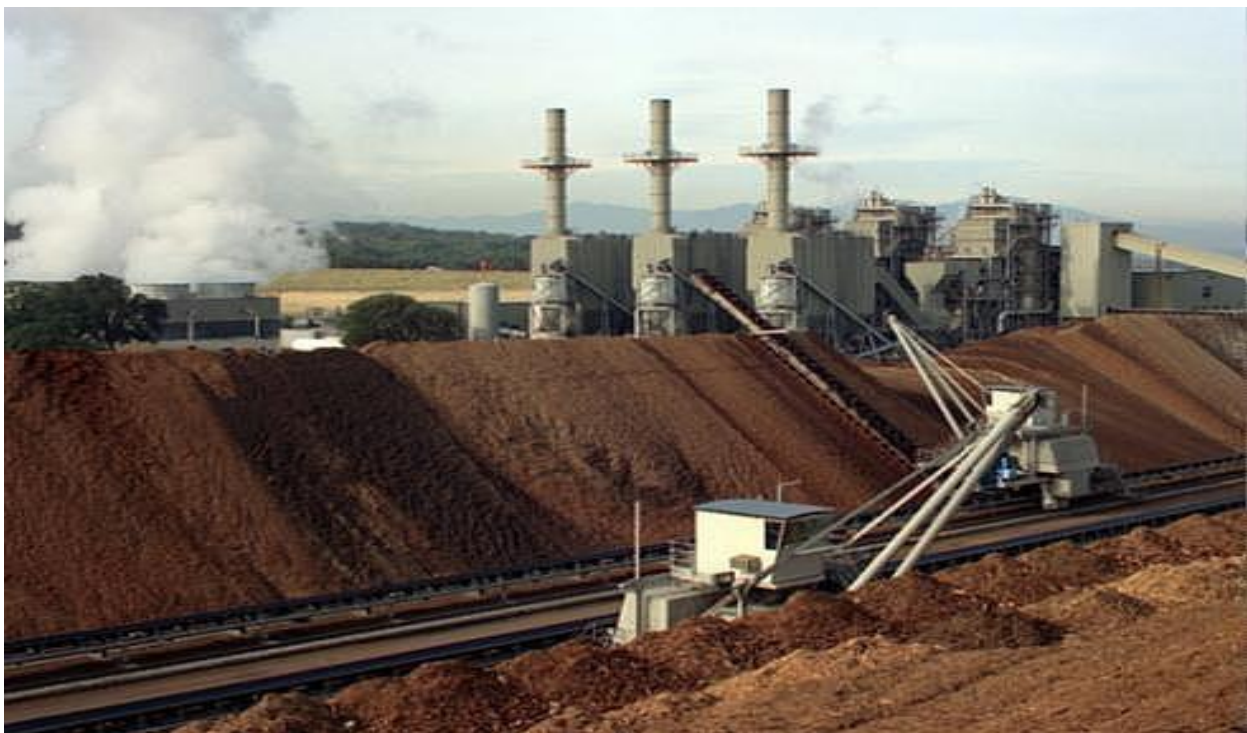
Figure 2.4: Biomass power plant
