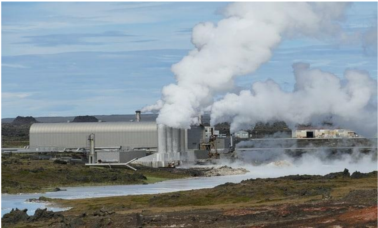
Figure 2.5: Geothermal Energy power plant
