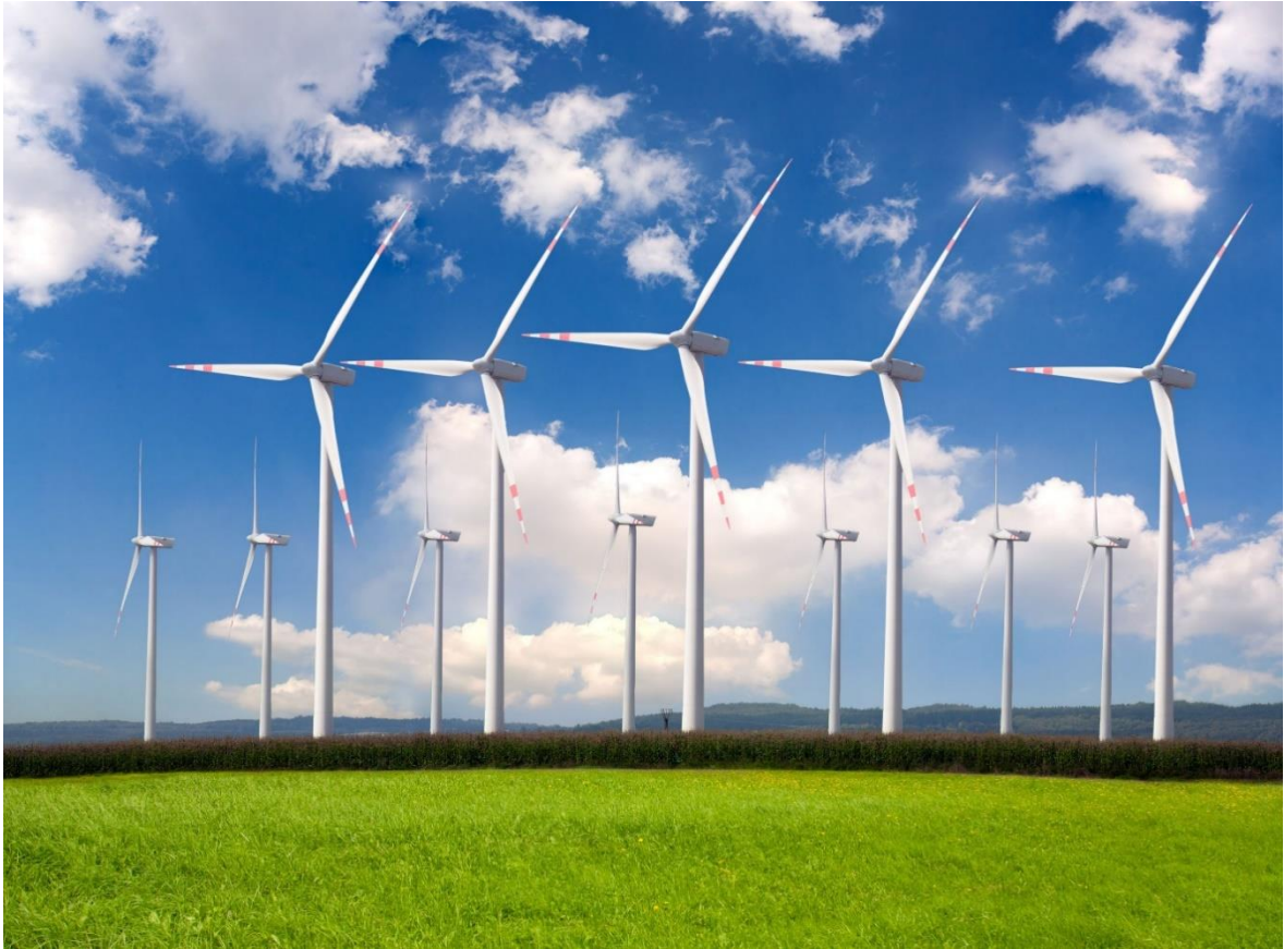
Figure 2.3: Wind power plant
