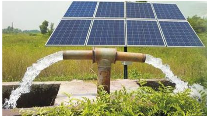
Figure. 2.17 Using irrigation of solar pumping system.
