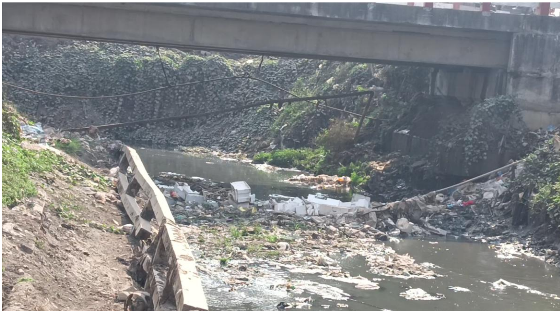
Figure 3.11: Unstable Terrain at Gabtoli Road
