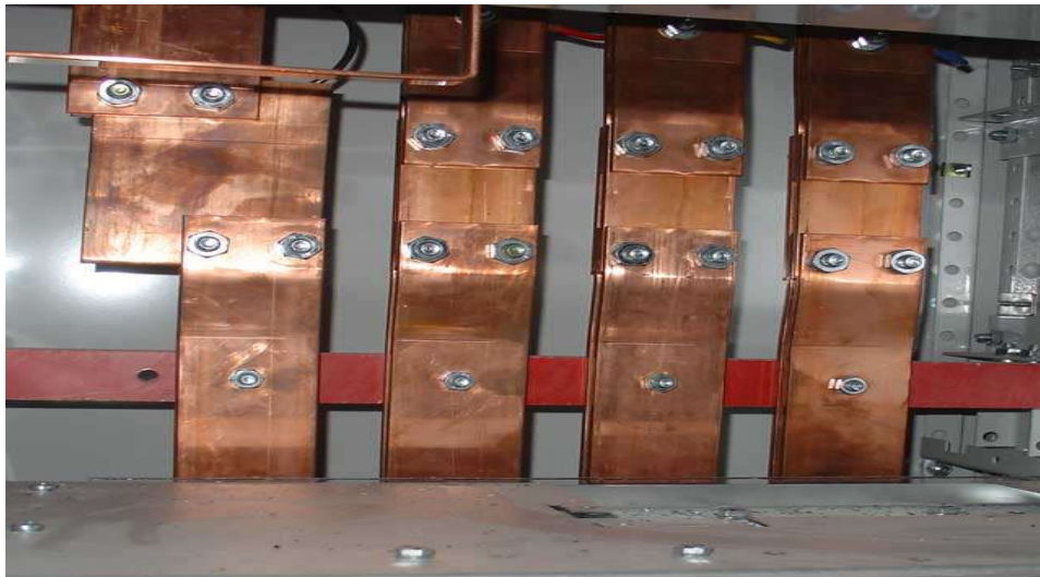
Figure: 3.7: Bus bar
