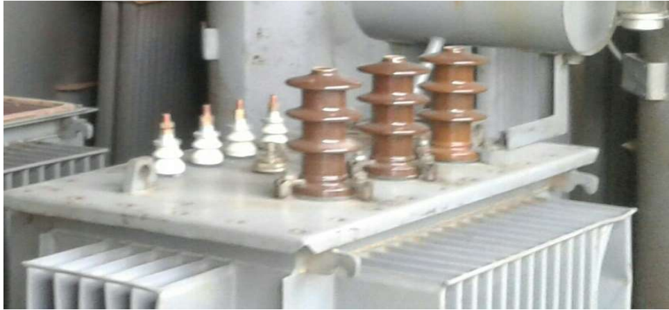
Figure: 3.14: LT and HT Bushing
