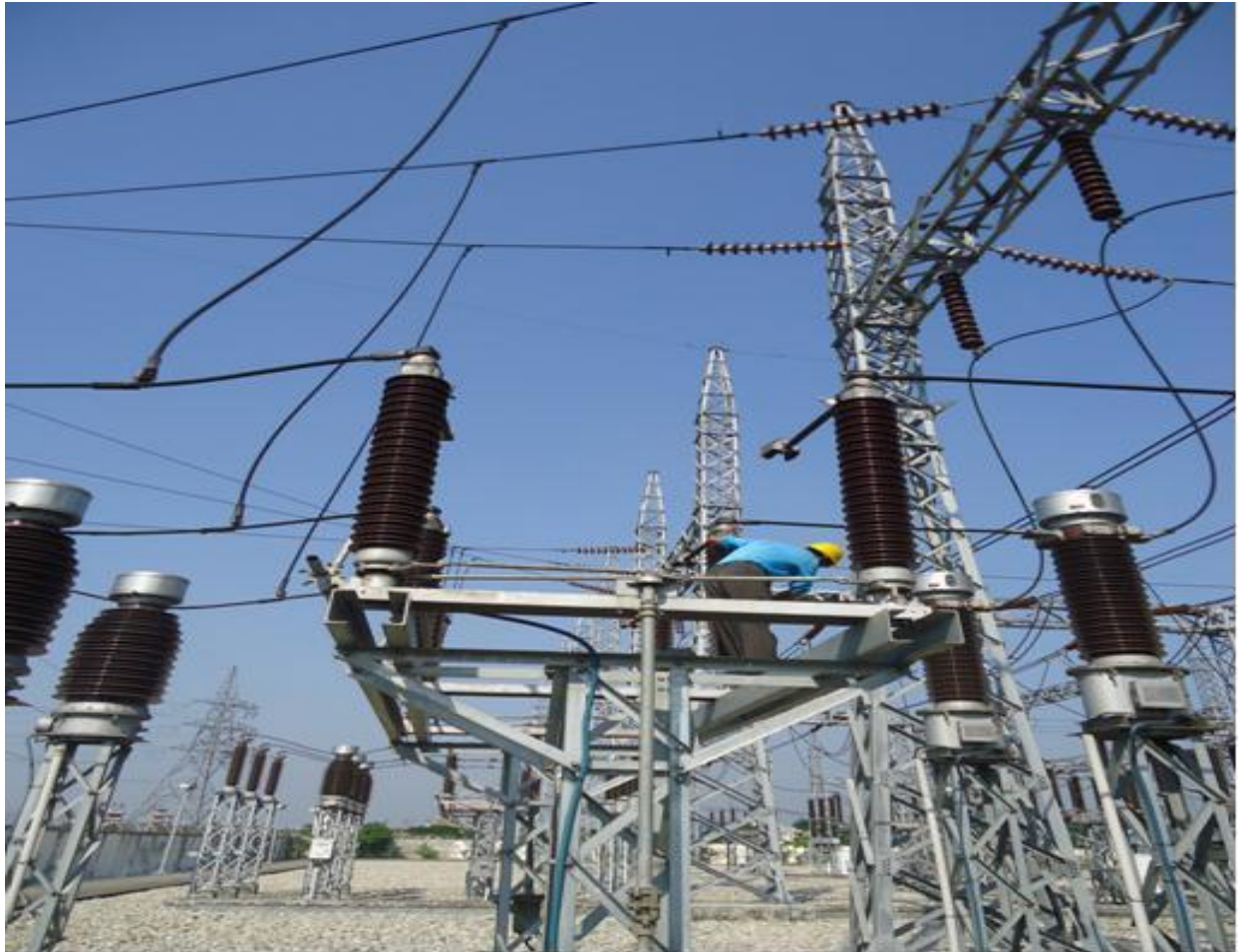
Figure-3.3 Isolation Transformer
