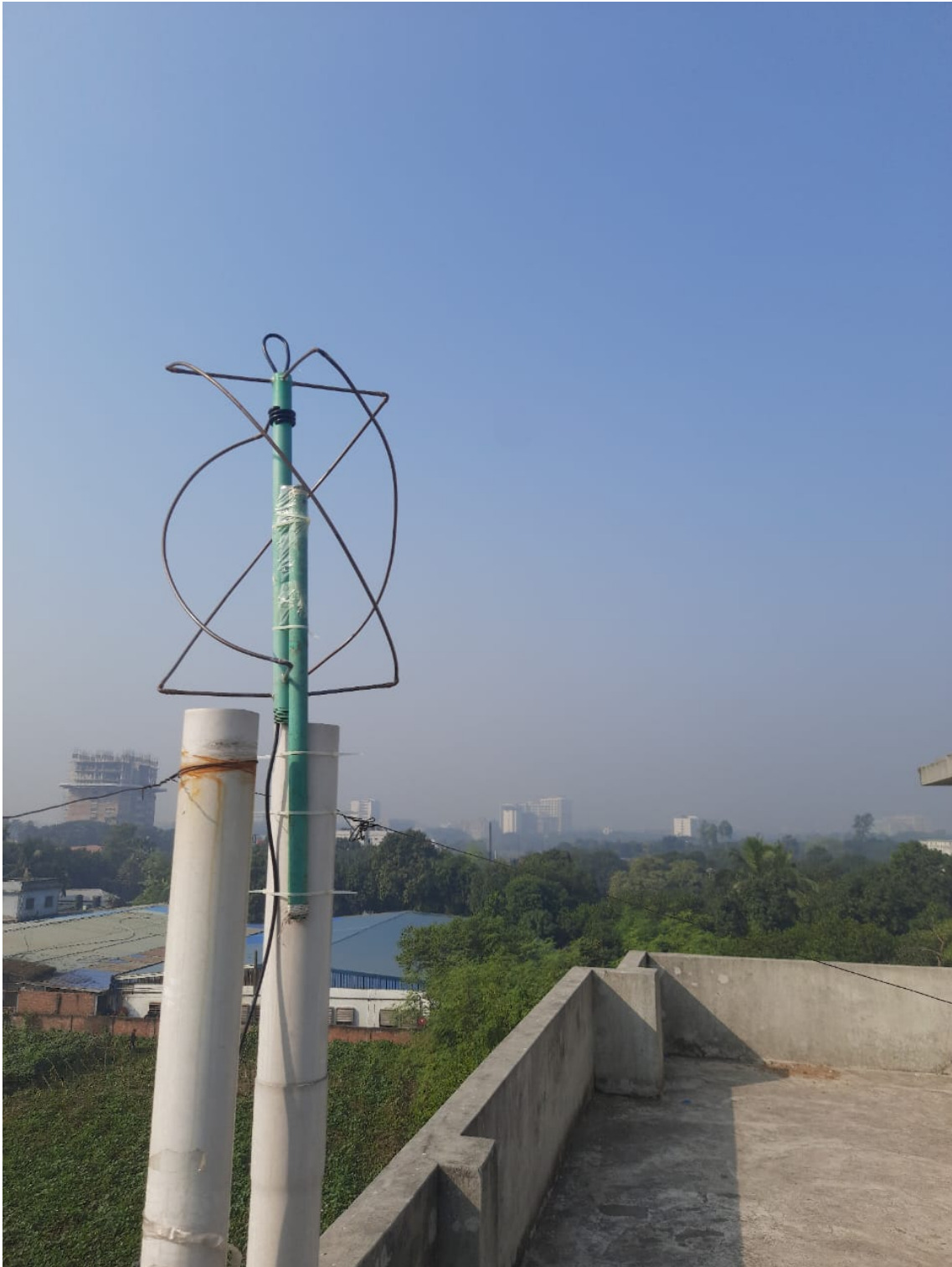
Figure 4.2: Final view of QFH Antenna
