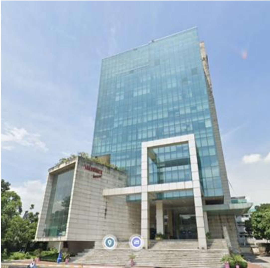
Fig: 3.5.1 Building Name: Anaya Tower
