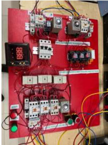
Figure 4.4: Phase failure Condition
