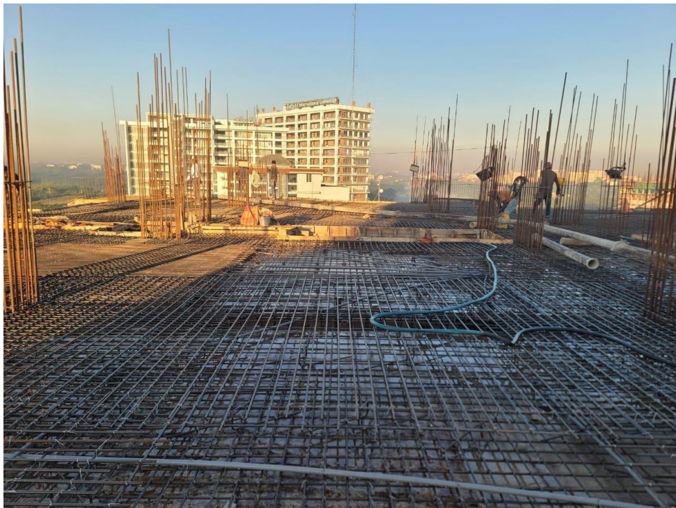
Fig. 2.4: Slab Reinforcement
